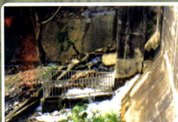
Crack and leakage at right side of the gravity dam.
