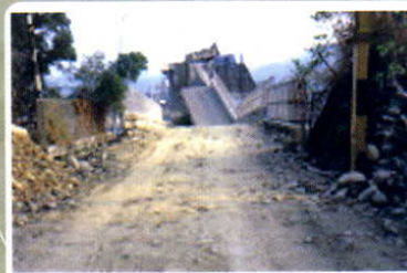
The wall at the right wing of the Dam was destroyed.
