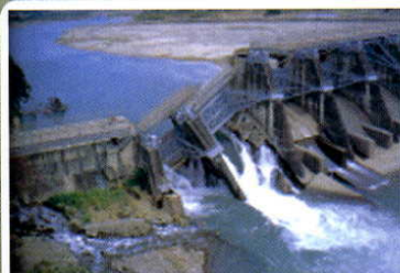
Damage at the right wing downstream face of the Dam (Spillways Nos. 16, 17 and 18 were severely damaged).
