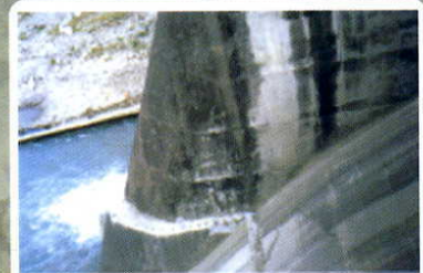
The pier of Spillway No.16, was broken.
