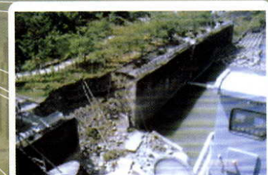
The retaining wall on the left wing of No. 1 sluiceway was damaged.
