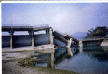
Spillways Nos. 16, 17 and 18 were severely damaged.
